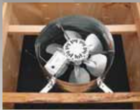
Exhaust Fan with Thermostat (mounts inside cupola)
